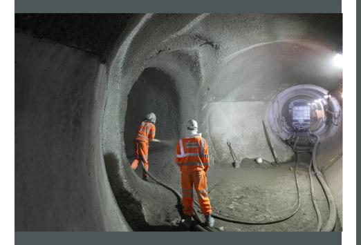
Supply and labour plant and materials to excavate and construct sprayed concrete enlargements within existing 2.85m ID tunnel. Two enlargements up to 6metre diameter were formed one for launching of TBM.
